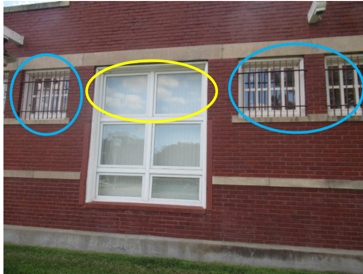
The historical design of the windows is circled in blue. All new windows (circled yellow) should be built to match.
