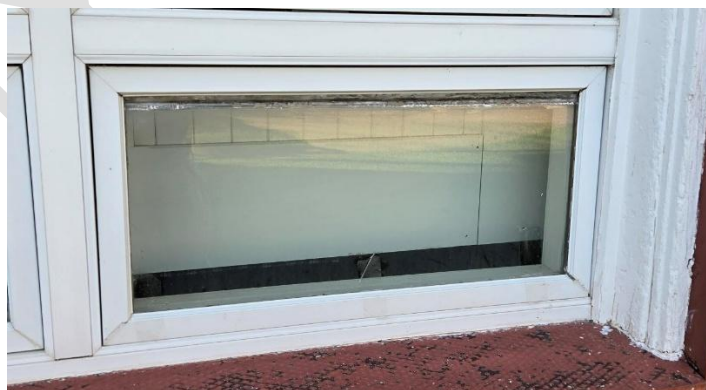
West window glass dropped within frame.
